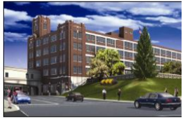
TK Budd Facility Redevelopment Revitalization
